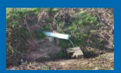
Subsurface tile drains intercept and collect shallow GW at the top of the water table which is discharged directly to the ditches.
